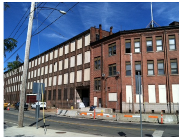
Construction is underway on the Winchester Arms factory (below.)
